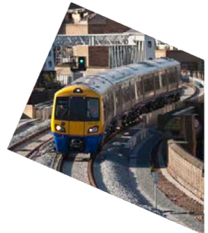
East London line extension
